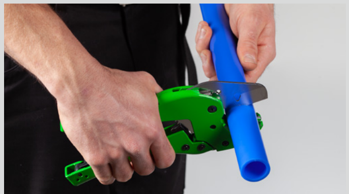
Cutting of the pipe
