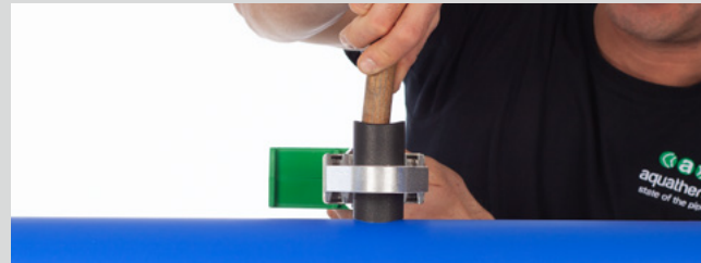
The welding tool is inserted into the pipe wall ...
