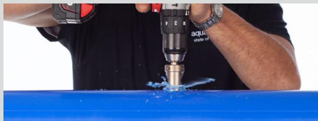
Drilling through the pipe wall
