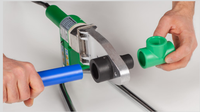
Heating-up of pipe and fitting
