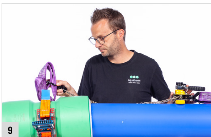
9 Attach the alignment tool securely to the pipe and the push-fit fitting.
