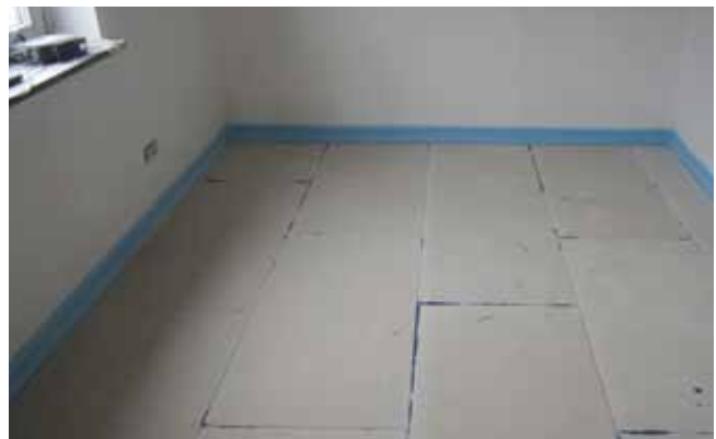
Finished dry elements
