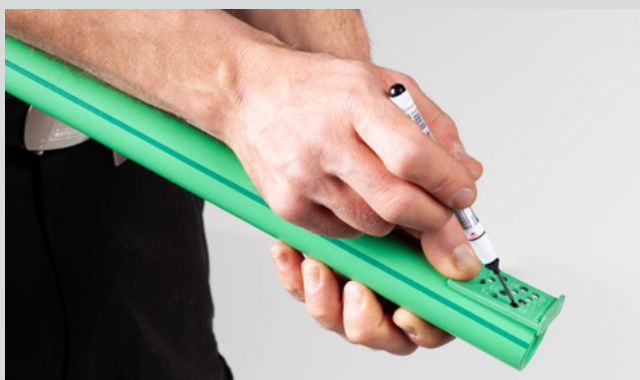
Marking of the welding depth
