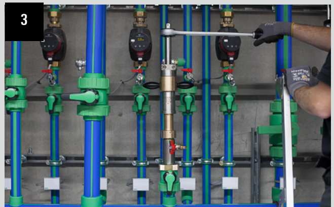
3. Start of the drilling process
