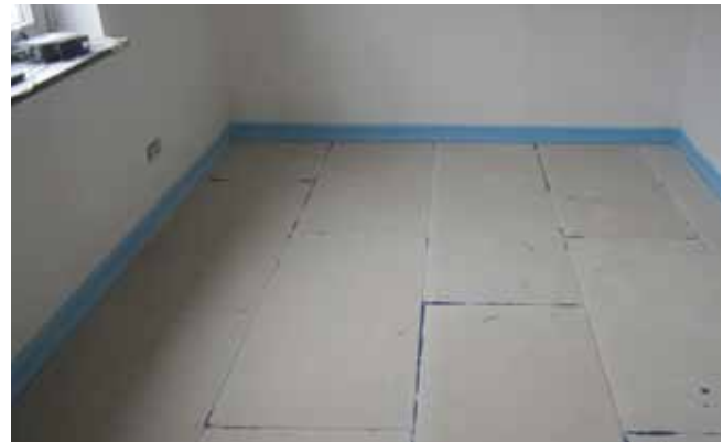
Finished dry elements
