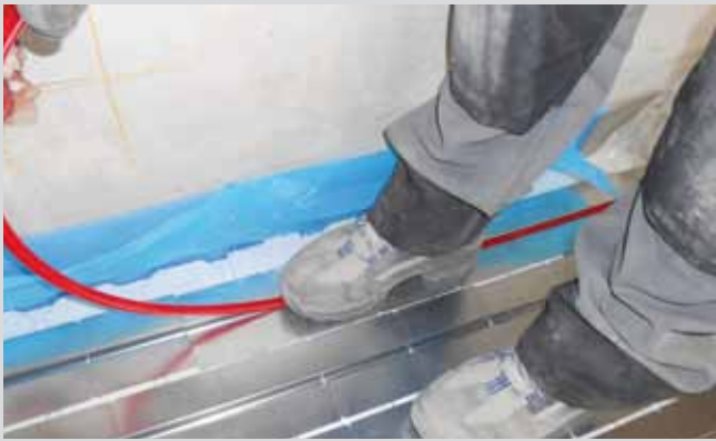
Laying of heating pipes
