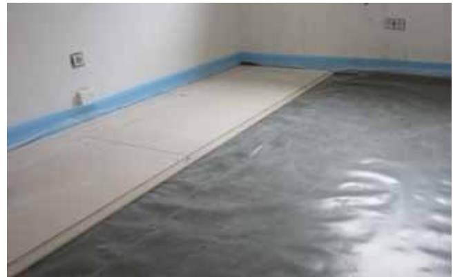
Before installation of the dry elements a release film made of PE is laid.
