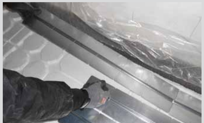
Installation of heat conducting steel sheets
