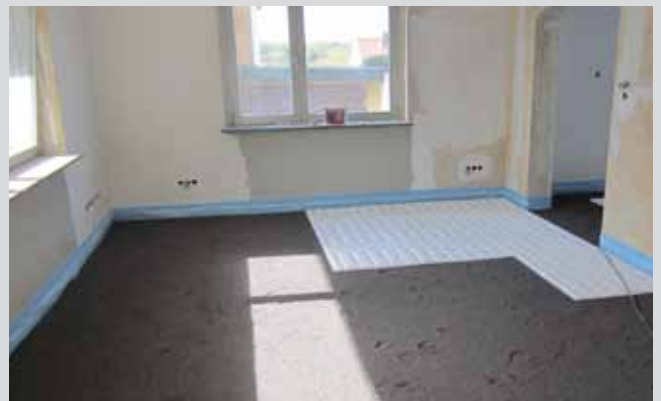
Laying of system element
