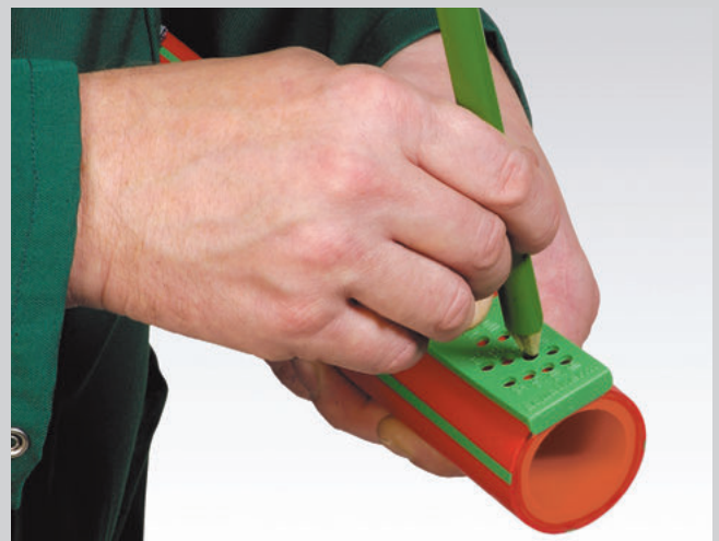
Marking of the welding depth
