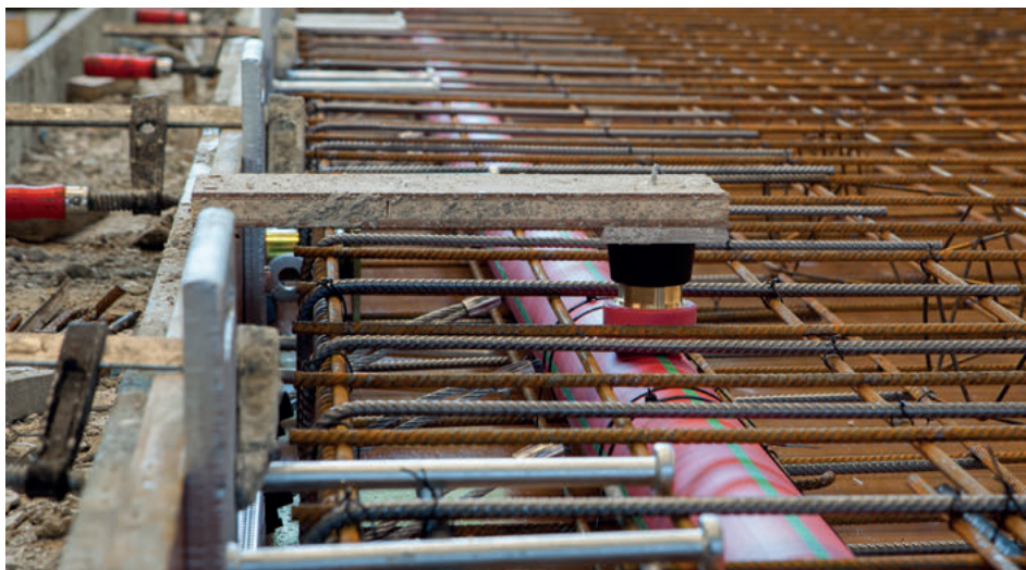
Prefabrication concrete wall
