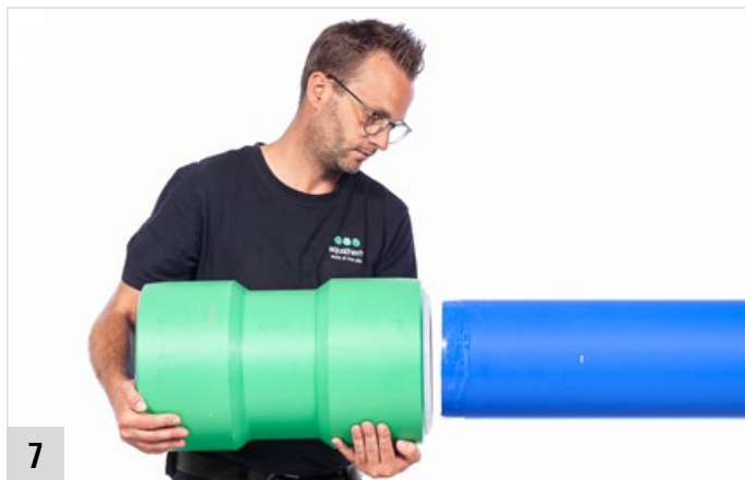
7 Place the push-fit fitting on the pipe end and press it over the first rubber seal.
