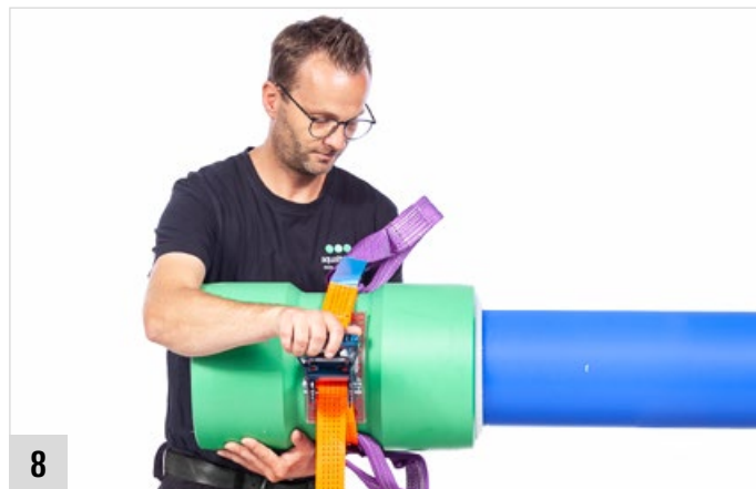
8 Final insertion of the pipe into the fitting must be done with an alignment tool.
