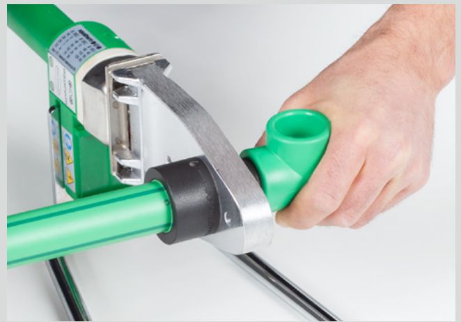
Heating-up of pipe and fitting
