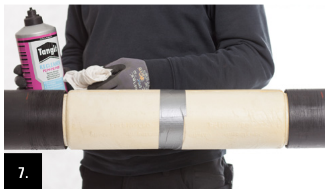
7. Clean sanding surfaces on both ends of the casing pipes with Tangit cleaning cloths or ethanol / spirit (at least 99.9%) and a dry, lint-free cloth.
