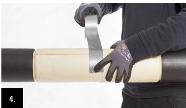
4. Fix the PUR insulation shells in the middle by circulating adhesive tape.
