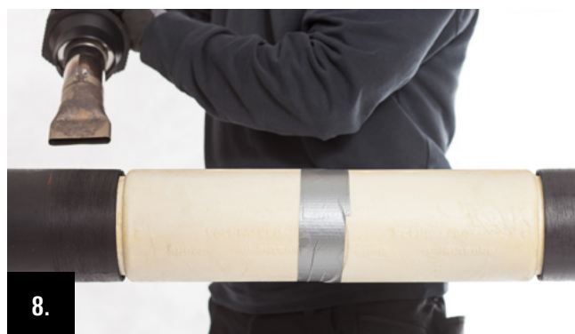
8. Attaching the shrink film: Heat cleaned casing pipe ends (with a soft flame when using a propane gas burner) to approx. 80 ° C. Check the temperature before installing the shrink film.
