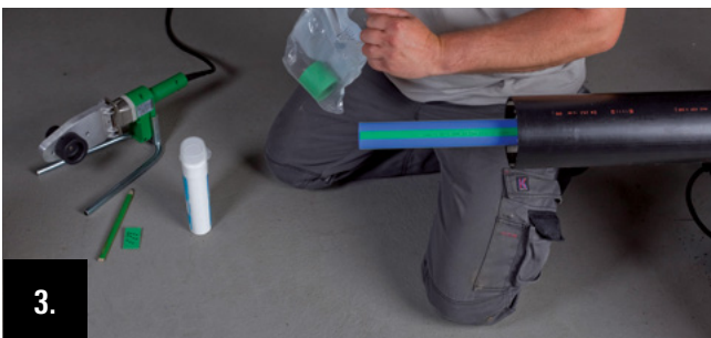
Take the aquatherm socket out of the packing. Loose fittings must be cleaned.
