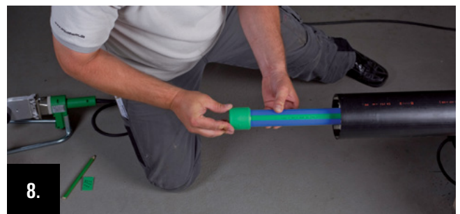
Align and momentary fix the welding socket. Further processing is carried out after the specified cooling time.
