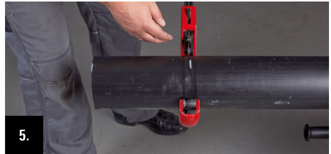
5. Cut the casing pipe with the pipe cutter up to the PUR-insulation layer around the whole pipe.
