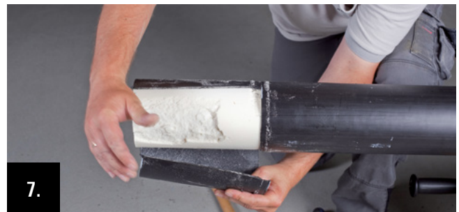
7. Detach the end of the casing pipe and then remove the PUR-insulation layer mechanically on the full skinning length.
