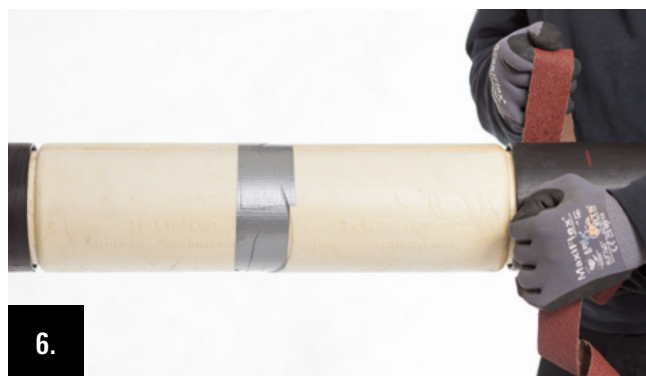
6. Preparation of the sealing area: Roughen the ends of the casing pipe up to the marking with sanding belt or abrasive cloth (grain size 40 or 60) over the entire surface and all around.
