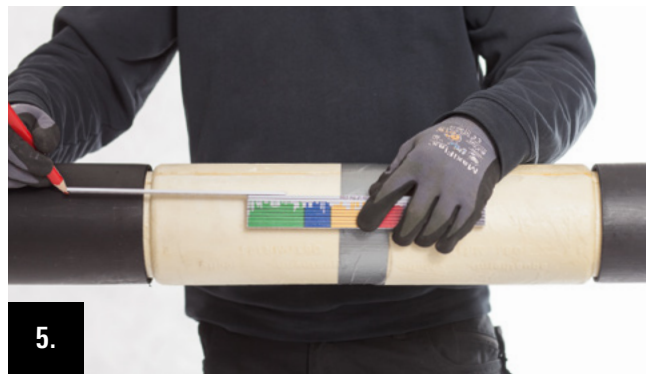
5. Marking the shrink sleeve position: To ensure uniform overlap of the shrink sleeve on each side, mark 30 cm from the center of the sleeve area.
