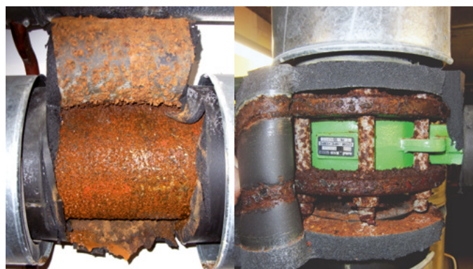
corroded steel pipes
