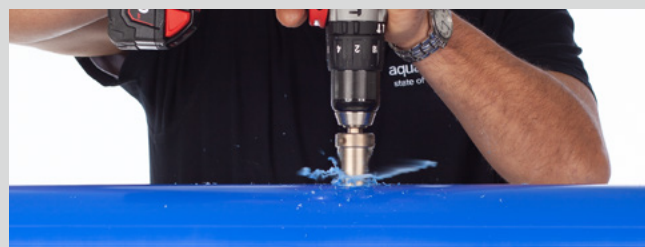
Drilling through the pipe wall
