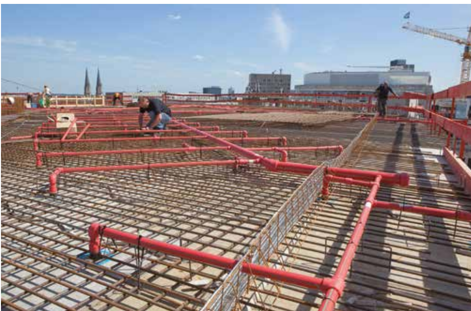
aquatherm red pipe Installation in concrete, Kö-Bogen, Düsseldorf
