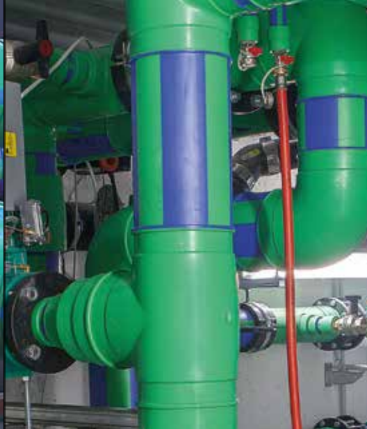
Welded connection PP-R
