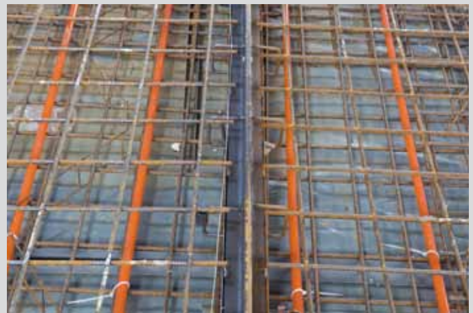
Preparation of construction joints by means of vertically adjustable seam joints
