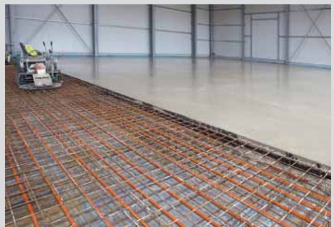
The surface is treated with a trowel
