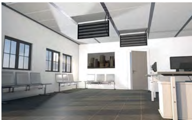
METAL PANEL CEILING AS STRIP GRID SYSTEM
