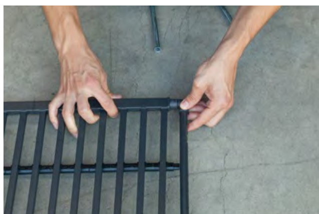
4. ... and push them together immediately (welding depth 13 mm)
