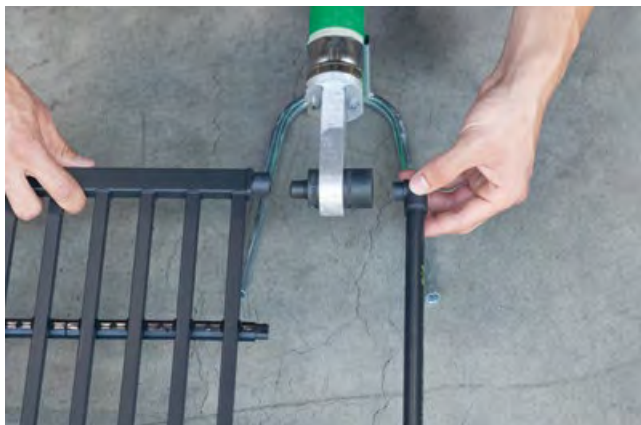
1. Welding device and tool (16 mm) are mounted; temperature control is performed.
