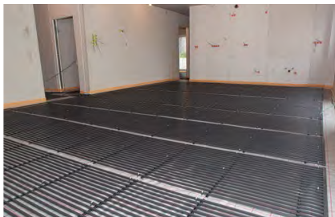
2. aquatherm black system as surface heating system on insulation at site.
